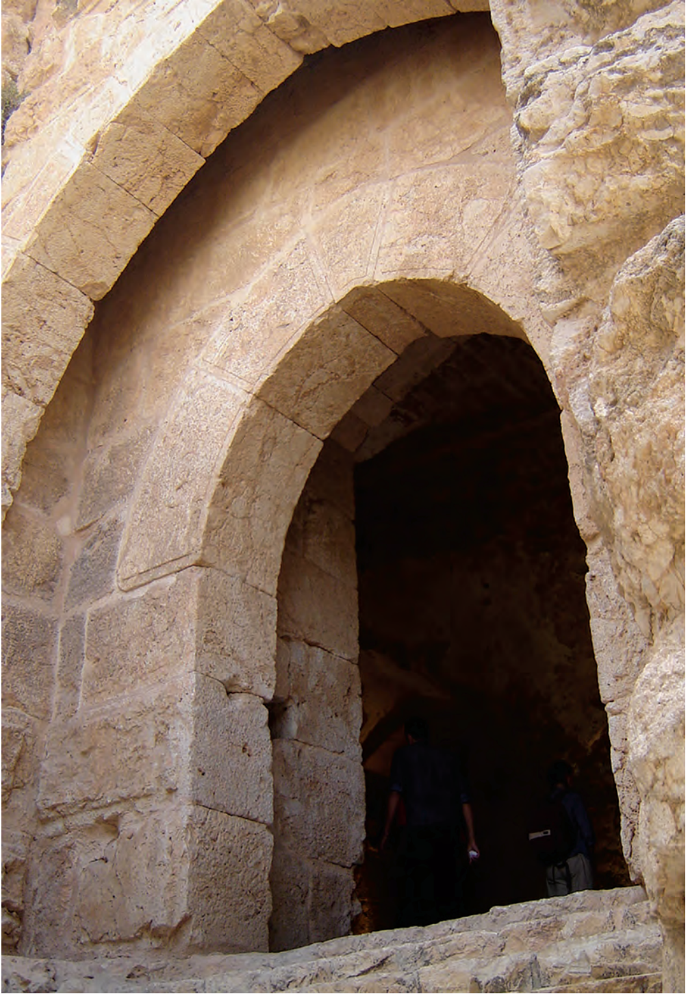
'Ajlun, slot machicolation over the inner gate of the outer gateway. (Michael Fulton)
